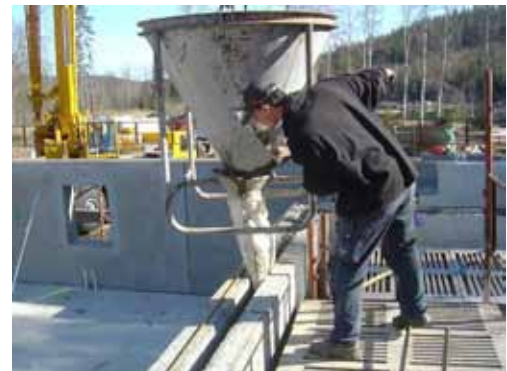
Figure 18 - Pouring of concrete
