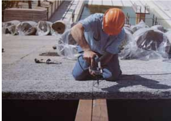
Figure 4 - Reinforced roofing boards (WWCB)
