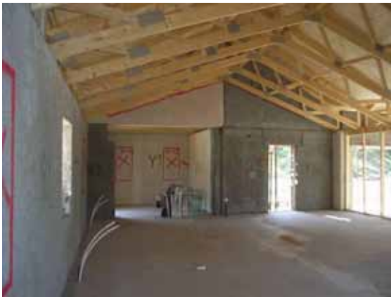
Figure 19 – Inner walls prior to stuccoing
