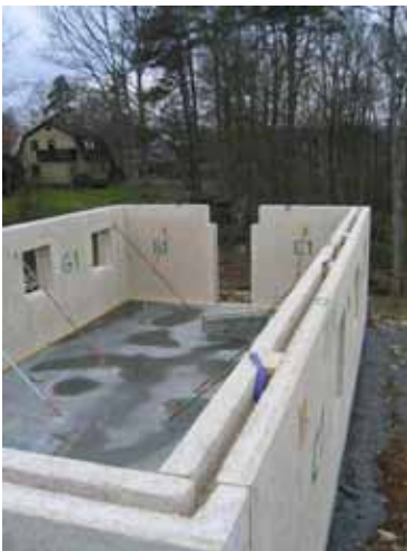
Figure 16 - Open Ring- beam
