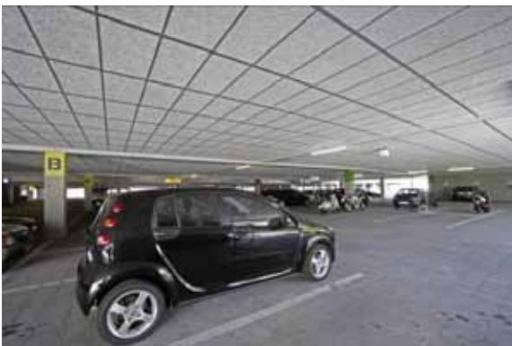
Figure 5 - Acoustic ceiling panels (WWCB)
